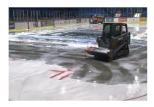
Pulling the ice partially with the ice resurfacer and then using bucket equipped removal apparatus is the most common method used in the industry. Bucket equipment should only be used by highly skilled operators as dasherboard damage or surface scars from poor operation will not be easily repaired. Equipment borrowed from other departments or rented are often poorly tuned resulting in toxic indoor air quality. Be sure to test and monitor. The
